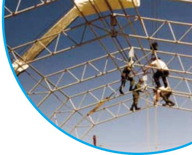
Typical truss framework for a Rubb structure
