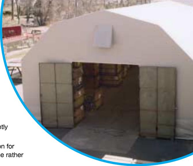
*Membrane replaced after 25 years - not because of age, but due to operational damage*
